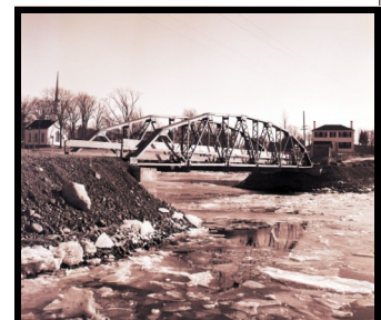
LITTLE DYERS RIVER BRIDGE 1952 SHEEPSCOT
