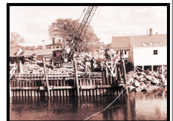
NEWCASTLE - DAMARISCOTTA 1952 BRIDGE CONSTRUCTION
